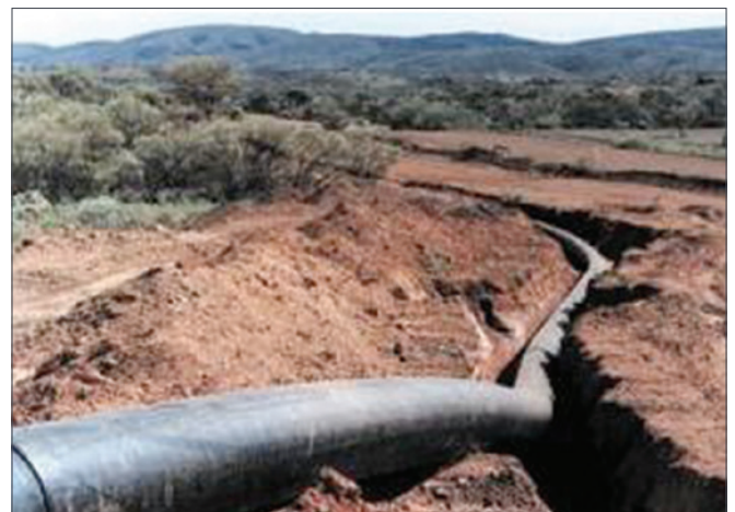
Figure 35b: In-field Laying of Multi-Jointed Pipe
